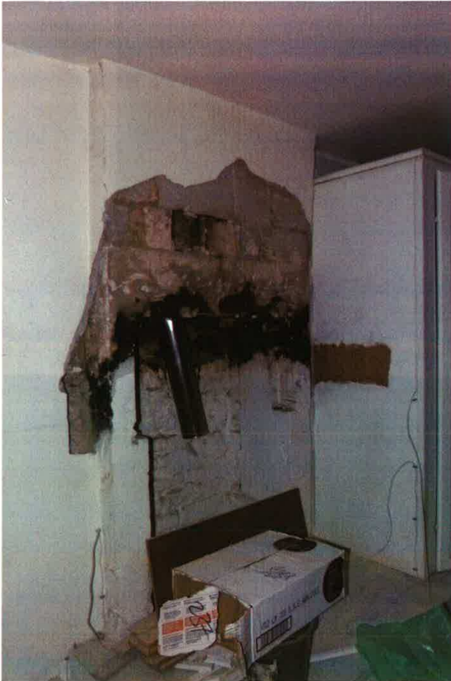
Room S6 – features removed
