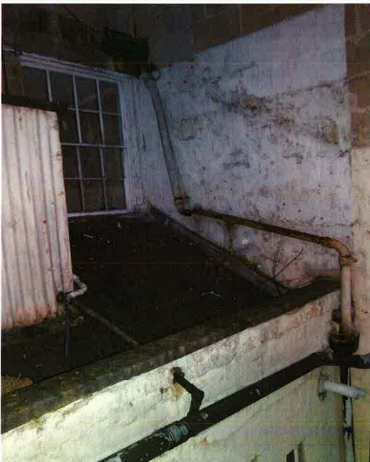
General condition of gutters and external area
