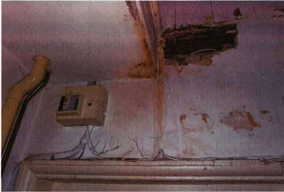
General Condition of building
