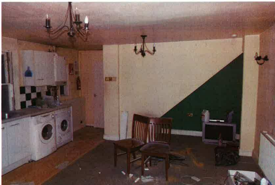
S1 – 20 th Century staircase to be removed.
