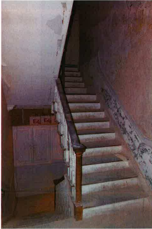
General Condition of Stairs
